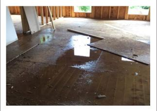
Because builders usually work on short, demanding schedules, and homes are being built tighter and more energy-efficient, the moisture introduced from the building process is not allowed to evaporate at the same rate it once did. The amount of moisture introduced during the building process can be significant. This moisture can be enough to create extensive flooring failures if not properly addressed.
